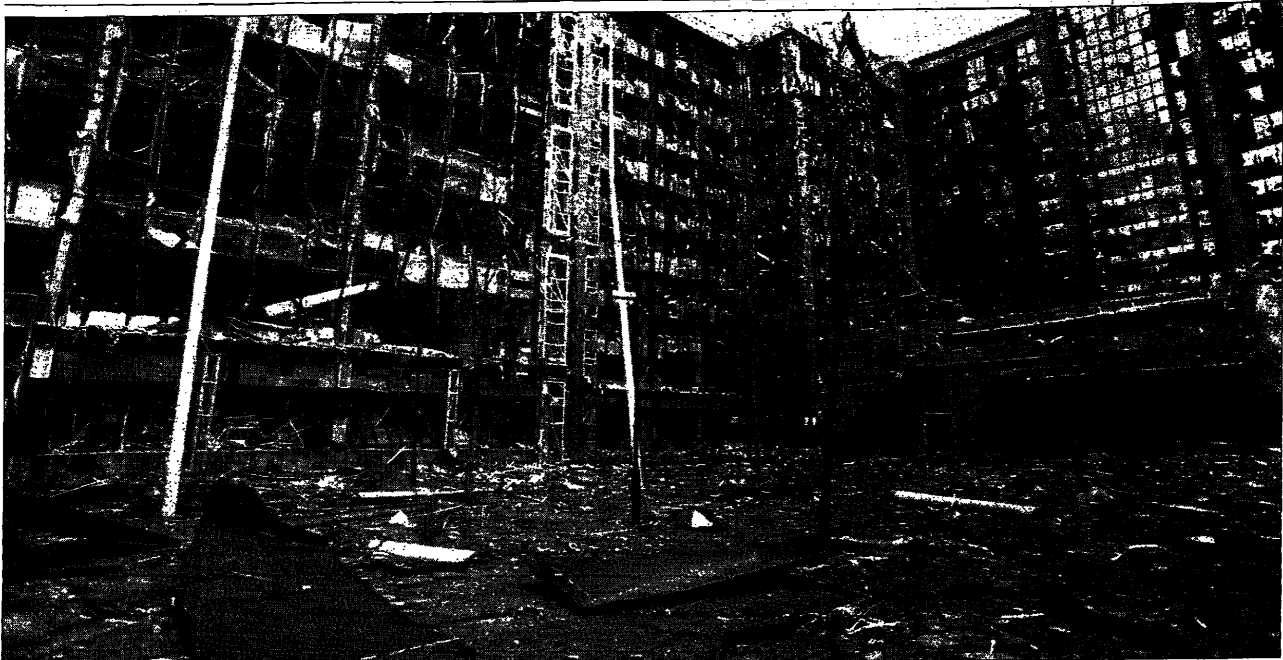
The dramatic aftermath of Friday's bomb at South Quay. Those assessing the damage say that although the buildings may look like skeletons with the windows blown out, their fabric may still be sound. PHOTOGRAPH BY DAVID SILLITOE
